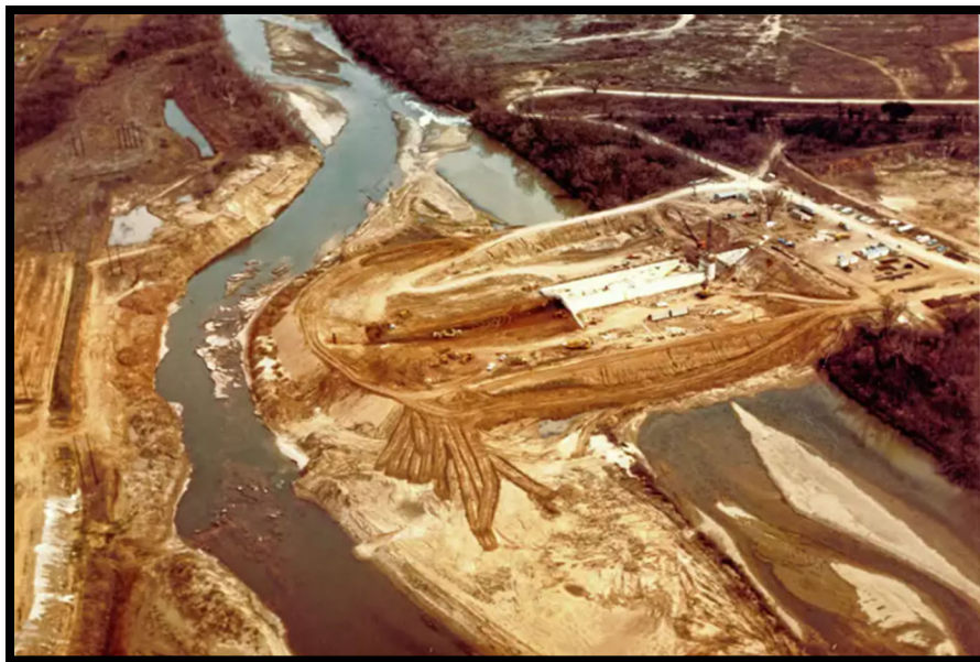
Construction of the Lake Brazos Dam in Waco, Texas.
