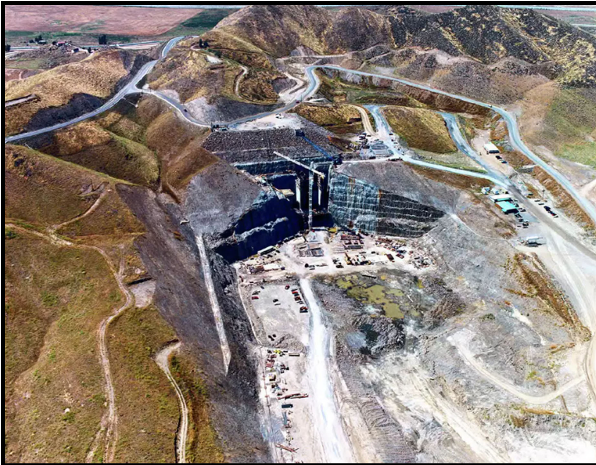
Construction of the West Dam in Southern California.
