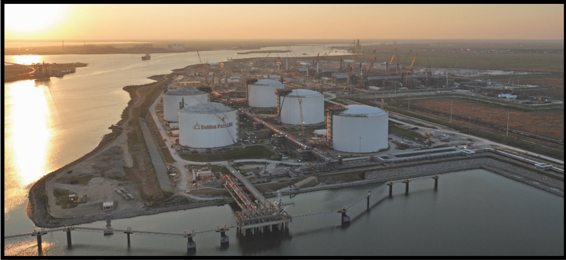
Construction of the GPX Project near Sabine Pass, Texas.
