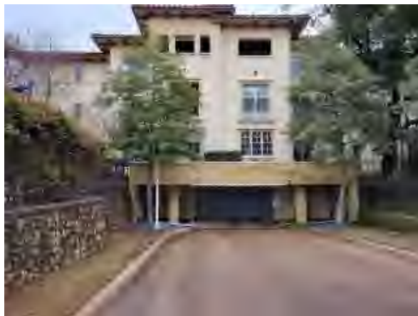
Williams #23 Wet wall, Building #8 Garage Entrance, west elevation at planter
