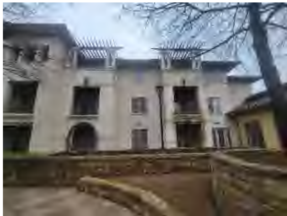
Williams #5 Wet wall, Building #1 PAC Courtyard
