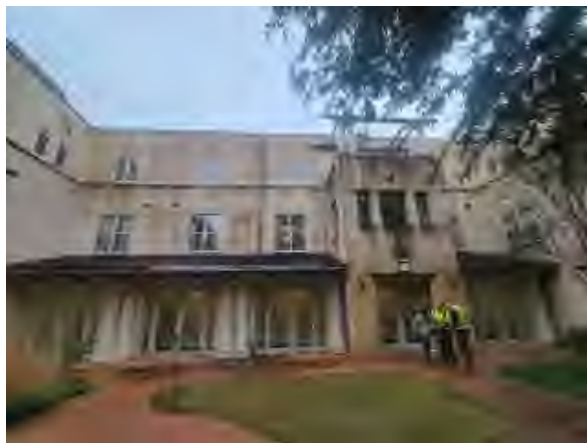
Williams #17 Wet walls, Plaza east courtyard
