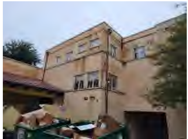
Williams #16 Wet Walls Plaza & Loading Dock
