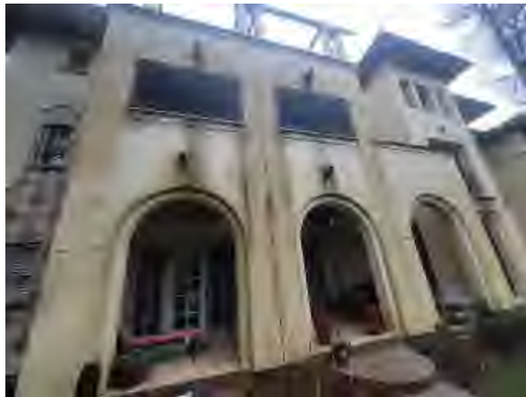
Williams #3 Wet wall, Building #2
