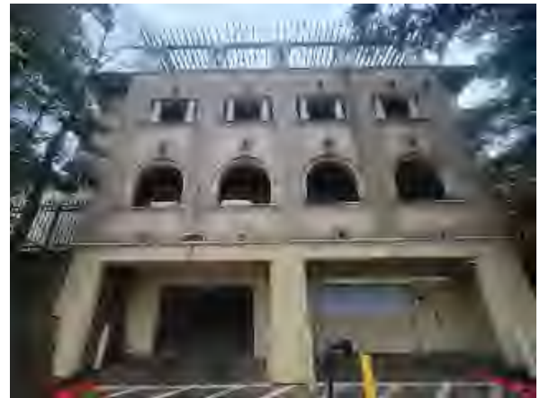
Williams #4 Wet wall, Building #3
