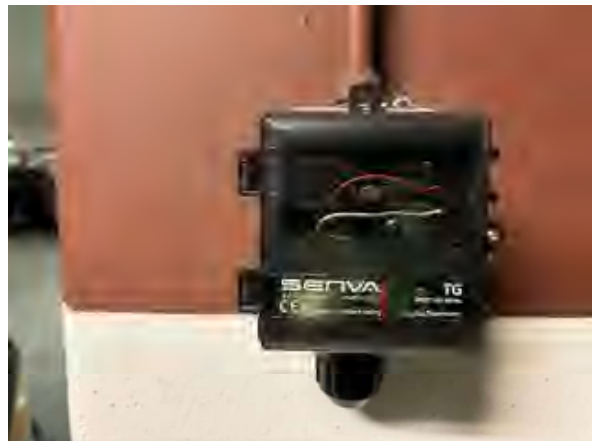
Freeman #12 Phase I Parking Area, Wall Mounted Toxic Gas Sensor. Not Operating (Continuation of #11)
