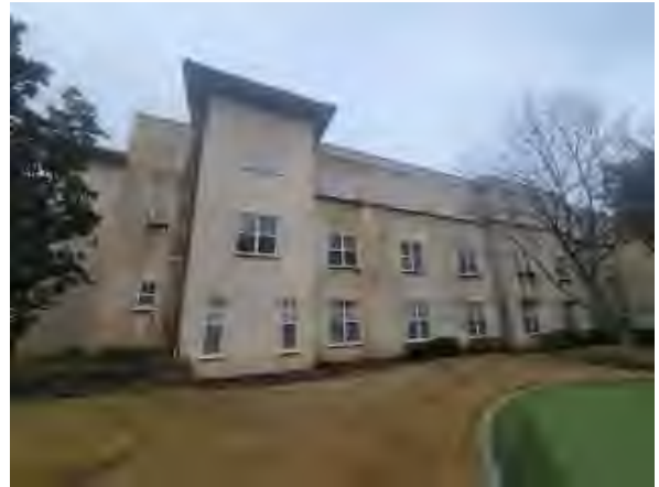
Williams #20 Wet Walls, Plaza Putting Green Courtyard, east elevation
