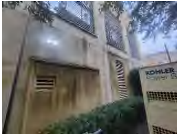
Williams #15 Wet Walls, Mechanical Room & Terrace (Chiller Enclosure) north elevation
