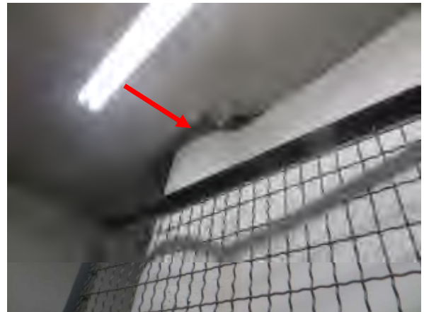
Flores #10 Storage area showing slab poured around existing pier. Note exposed rebar (arrow.)
