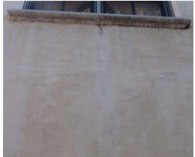
West Commons – Exterior Façade Cracking
